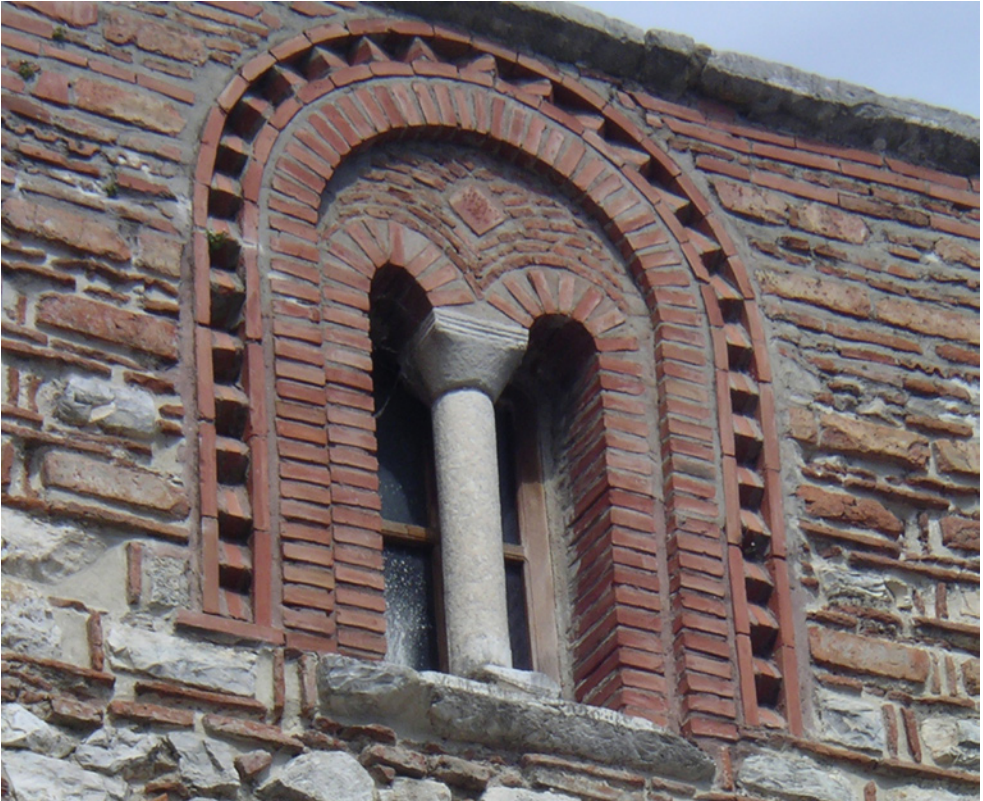
Fig. 50. Arta, Ag. Theodora. Detail of masonry in the S façade.
